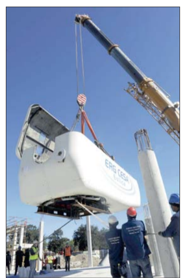
WIND POWER: Assembling a wind turbine at Cape Peninsula University of Technology. PICTURE: CINDY WAXA
